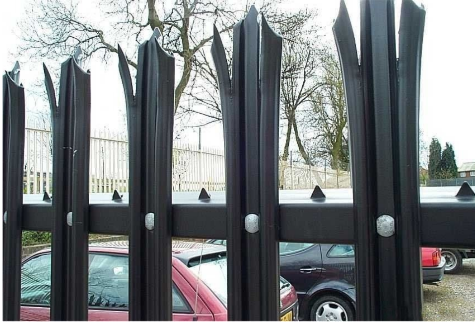
Profiled pales, protected fixings and anti-grab top rail
